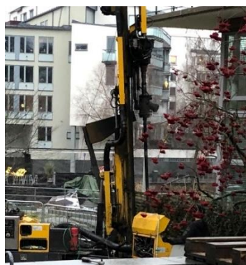
Borrning - Installation utmed Sickla Kanalgata
